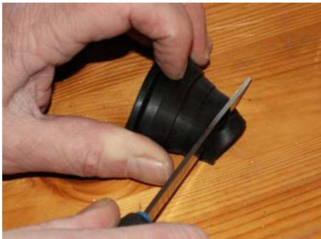
Drill a hole (dim 19 mm) in the appropriate place in the cabinet for cables. Mount the cable grommet seals included in the kit. Complete installation of the plaster-board wall (normally 13 mm gypsum). Make sure that the plaster-board does not end sit flush with the exterior of the cabinet; the cabinet's frame should "sit" on the plaster-board. (See the image below).
