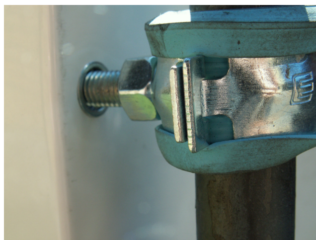
Close up on attachment to cabinet.
