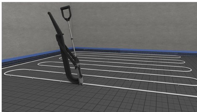
Attachment of pipes on LK Foil Board 30 Silent.
