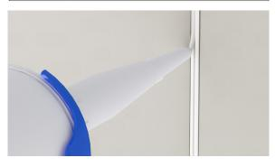
2. Seal and fill between wall and the hatch's outer frame.
