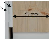
For certain installations such as the LK Manifold UNI-Avst (and the number of outlets in the cabinet will be reduced) or the Minishunt M60, the cabinet must be mounted 10 mm inside the stud frame, or alternatively a double plasterboard or a plasterboard and OSB board must be mounted on the stud frame.
