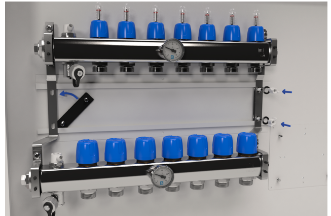
Installation of LK Manifold RF.
