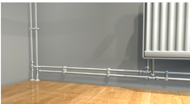
Example of clamping, visible installation
