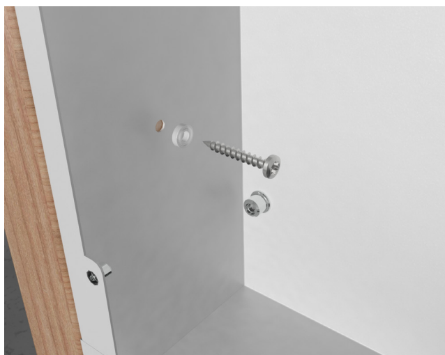
Attaching a cabinet to a stud wall.
