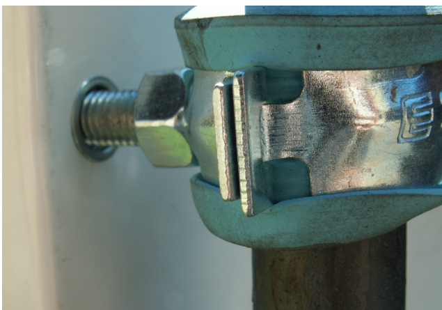
Close-up of fastening to cabinet.
