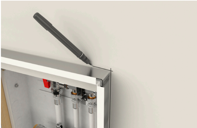
Mark the outside of the frame on the plaster board
