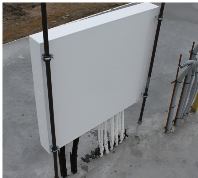
Installed cabinet stand.
