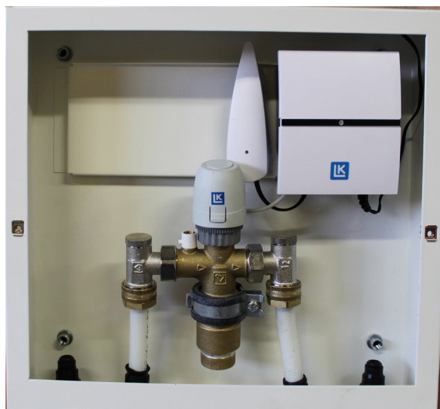
LK Mini Loop Valve M5 supplemented with LK ICS-RF1. The equipment is installed in LK Cabinet M5 WP-XL.
