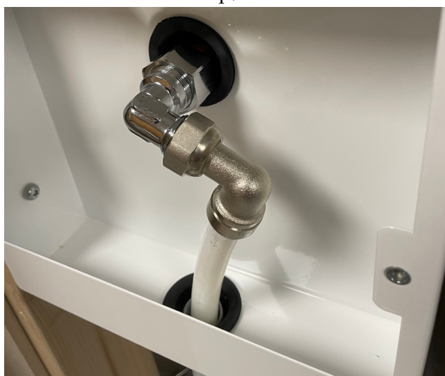
An example of an assembly that does not cause tension in the coupling.
