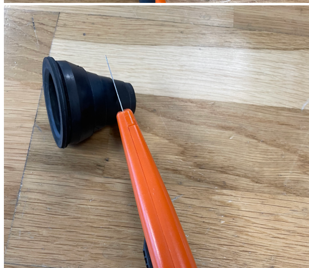
Cutting of a LK Pipe Inlet 20-25 LP. It must be adapted to the copper pipe of the outdoor tap/faucet.
