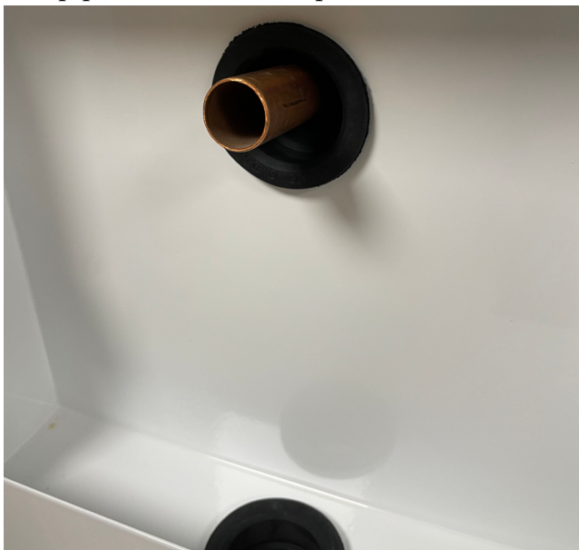
The inside of the cabinet with the pipe inlet and the copper pipe.
