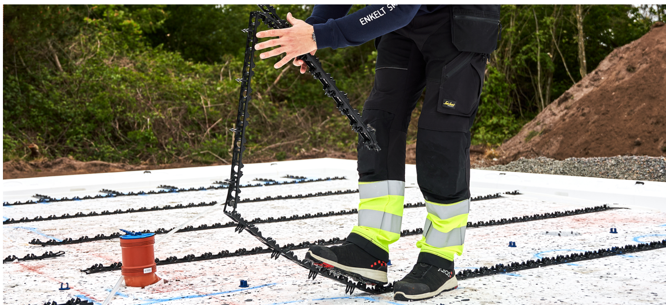
A fitter unfolds and inserts the rails in the EPS isolation.
