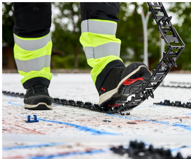
LK Clip Rail Combi 16/20 on EPS insulation.
