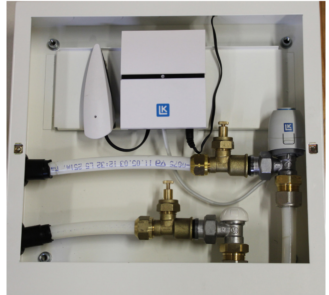
LK 1-Circuit Valve supplemented with LK Connection VKF RF/1-Circuit Valve Set and LK ICS-RF1. The equipment is installed in LK Cabinet M5 WP-XL.
