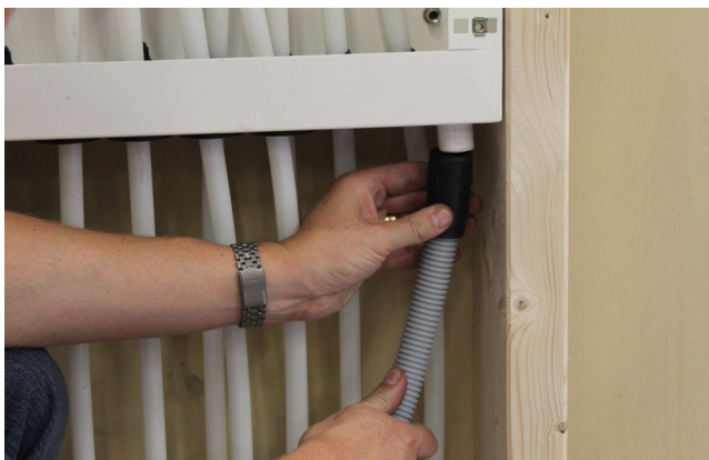
Assemble the rubber sleeve
