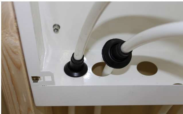
Fit the pipe grommets.
