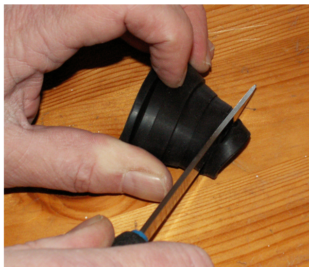
Cutting of a LK Pipe Inlet 20-25 LP.
