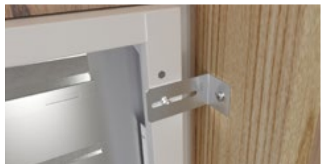
Angle brackets mounted before installation in building structure.
