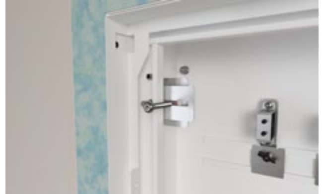
Installing the wet zone hatch in the cabinet.
